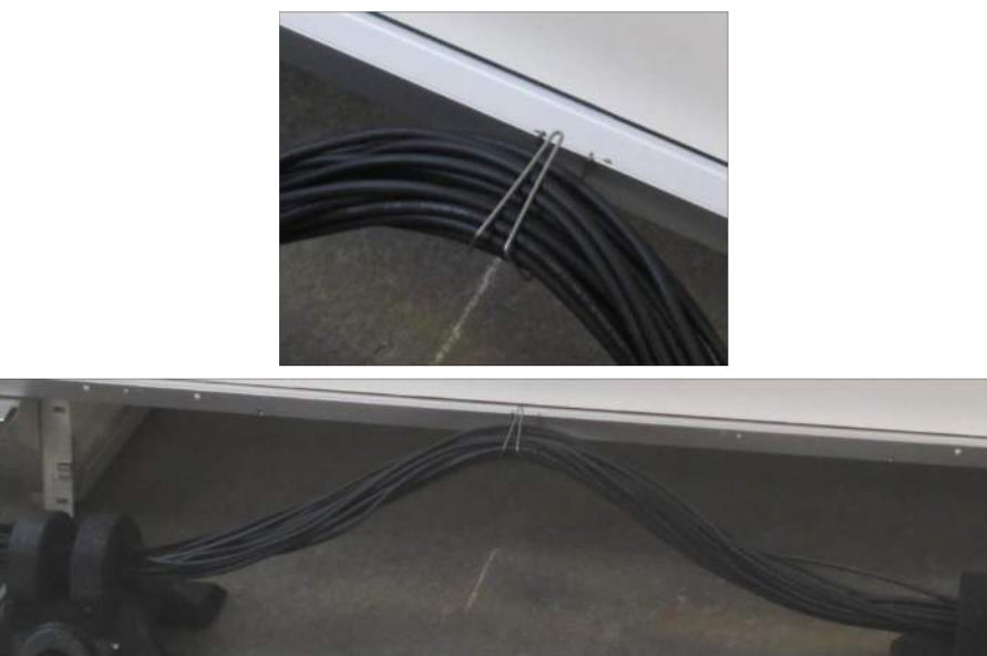
STEP C – SECURE HOMERUNS WITH WIREFORM CLIPS
