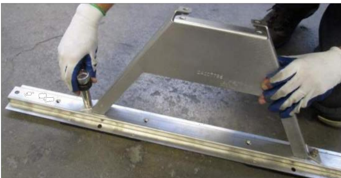
STEP A – INSTALL REAR LEG TO RAIL
