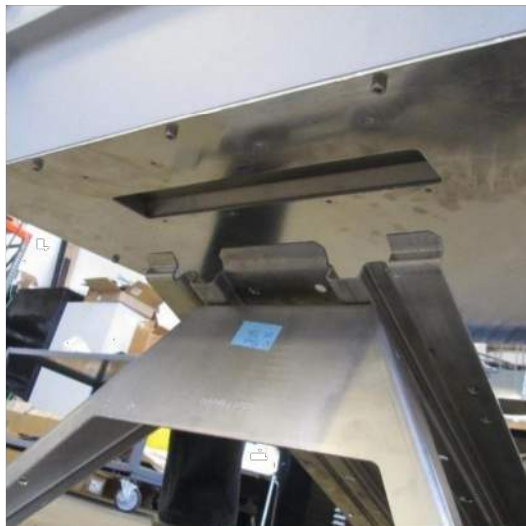
STEP B – ALIGN MOUNTING TAB WITH INVERTER SLOT
