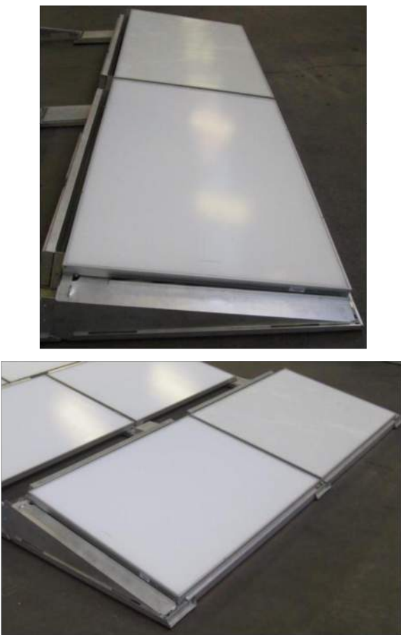
STEP D – COMPLETE MODULE INSTALLATION
