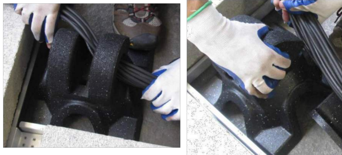
STEP A – ROUTE HOMERUNS THROUGH STUMPS
