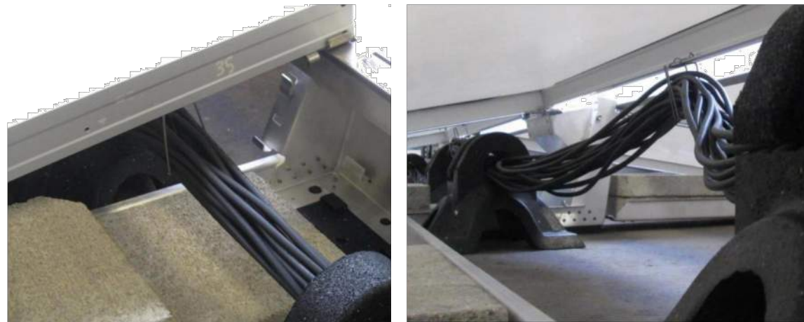
STEP A – SECURE MODULE-TO-MODULE WIRING
