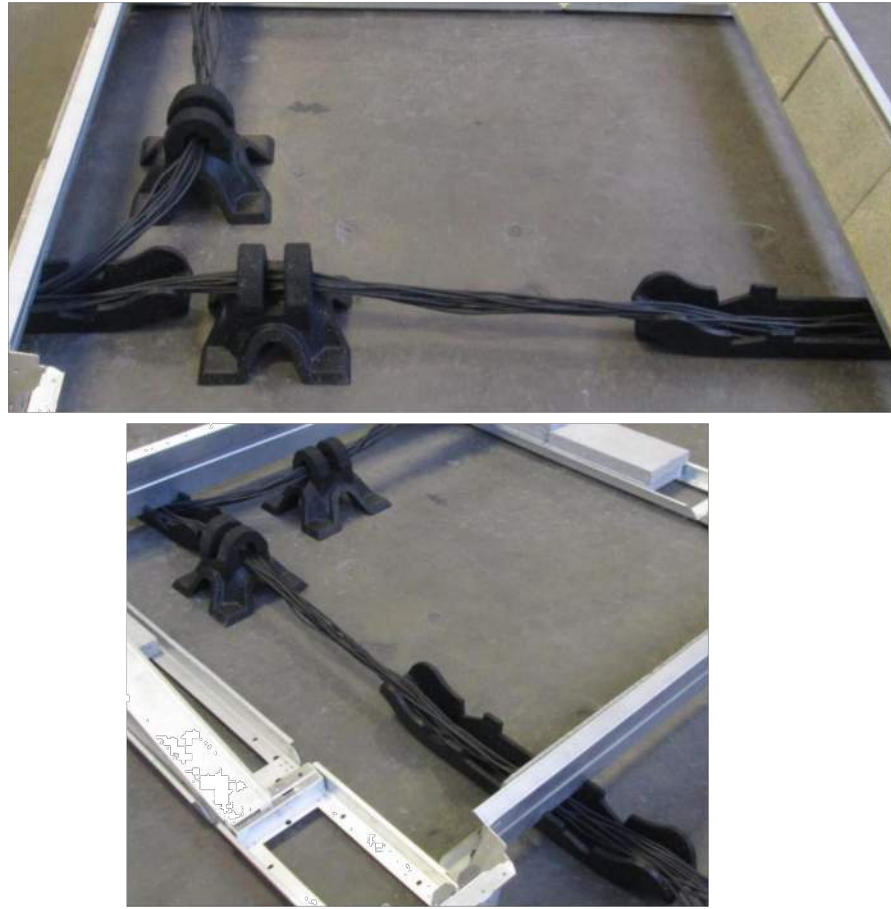
STEP D – ROUTE HOMERUNS N-S & E-W
