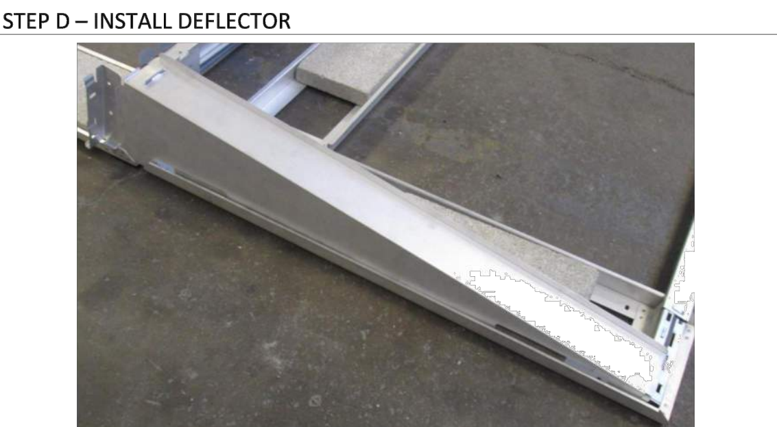
STEP D – INSTALL DEFLECTOR
